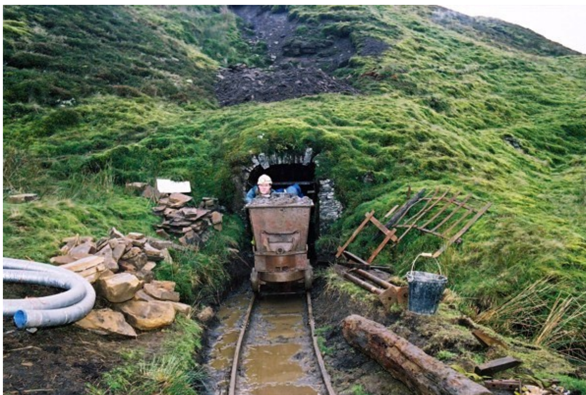
Conservation work at Middlecleugh mine
