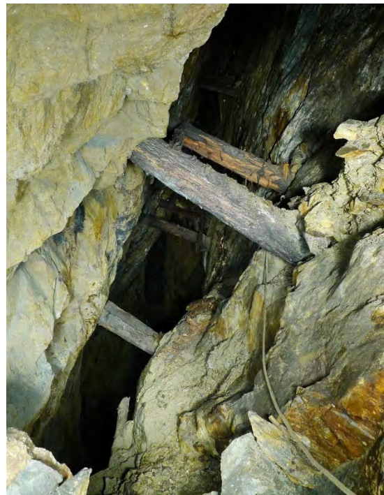
Photo 7 Missing floor very close to Thriddle Shaft
