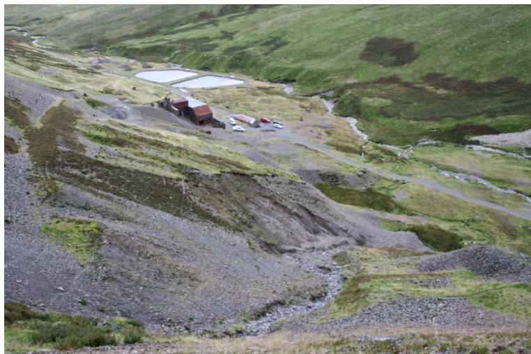
Force Crag Mine with the treatment plant using the original settling ponds.
