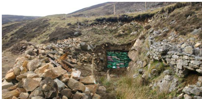
The portal left secure prior to installation of the bat friendly gate
