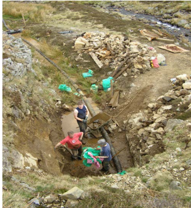
Andrew Woolard, Warren Allison and Rosemary Vidler working at the portal The water by-pass pipe and ponding dam can be seen.
