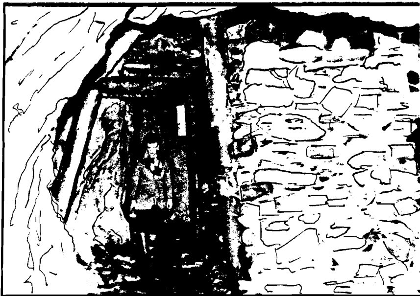
Shaw's timberwork by the side of the Old Engine Shaft in 1962 - put in during the c.1954 attempt to re-open the mine. The woodwork and packing is now collapsed. A large boulder fallen from the side lies over the ladderway. Efforts have been made to clear away some of the debris here.
