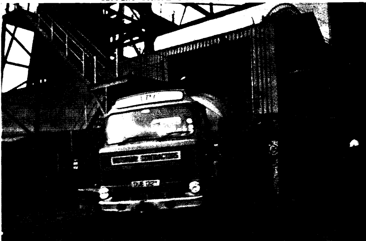
TIPPING CONCRETE DOWN No.5 SHAFT
