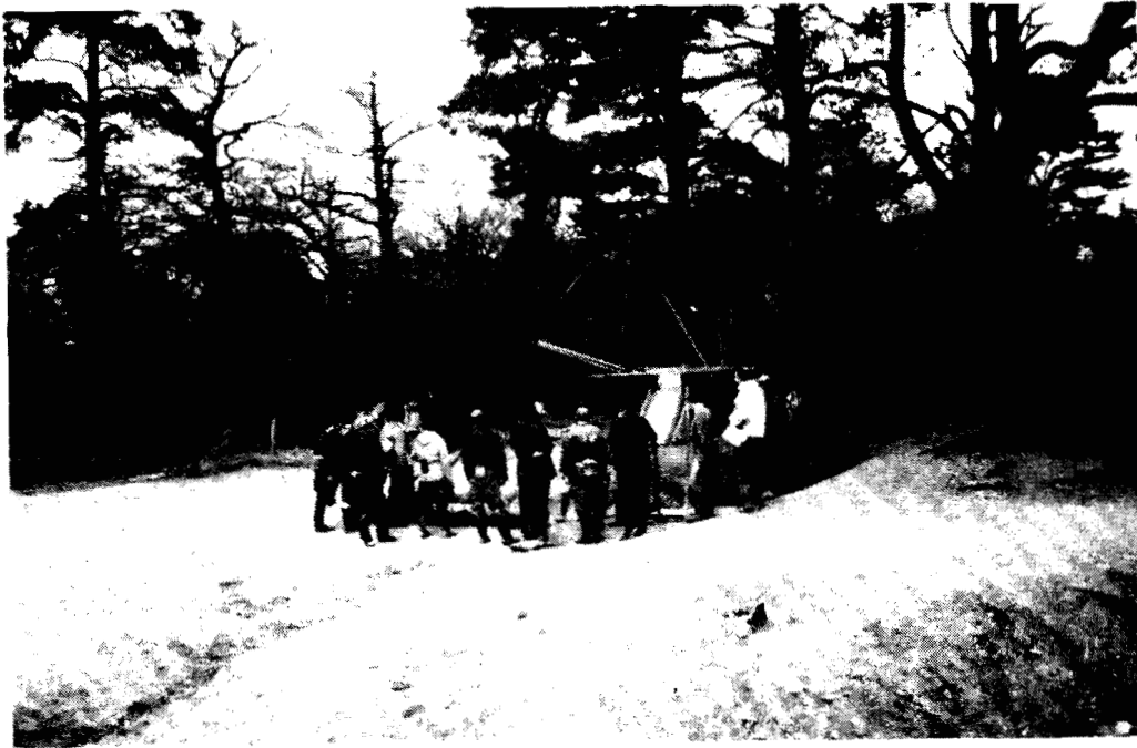
Photo; head gear on Bear Pit shaft, note trap door platform and spoil chute for tipping kibble spoil directly into waiting dumper truck.
