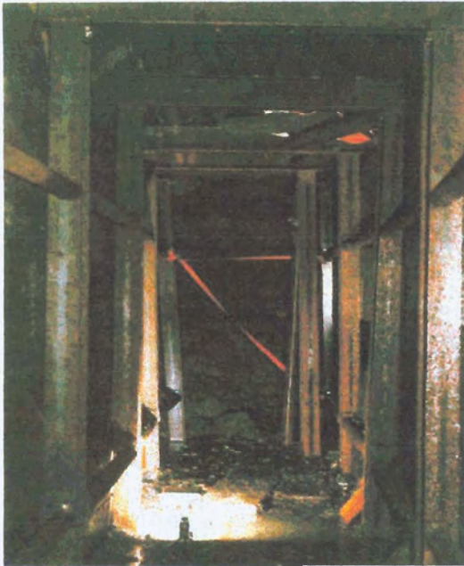
The first four frames in place. All of this space was completely filled with rubble.
