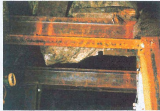
Detail showing one of the large boulders which was jacked up to rest on top of the steel work.
