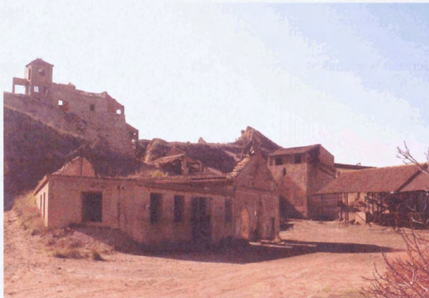
Abandoned mine near Cartagena. The tower on the skyline is at the top of a shaft, and still contains the headgear and cages. In other buildings there are shaking tables and classifiers.
