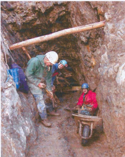
Preparing to erect the timber work
