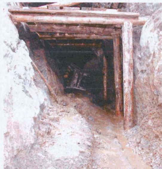
The remaining spoil will be dug out and piled on top of the timber frames. In due course material falling from the sides of the crater will cover it over
