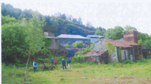
Backbarrow Furnace, showing the re-roofed barns behind the blast furnace and boiler. The horizontal steam engine is in the main foreground building. Molten iron was cast into pigs on the flat area to the right of the picture, but the casting house has long since been demolished.
