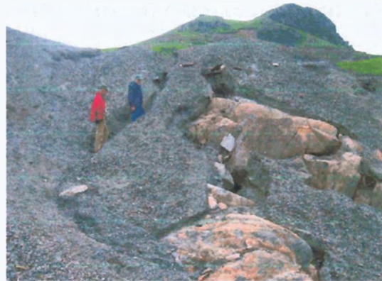
Water from a buried culvert has washed away part of a spoil heap.
