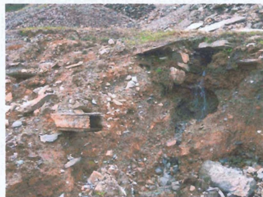
Wooden water trunking exposed.
