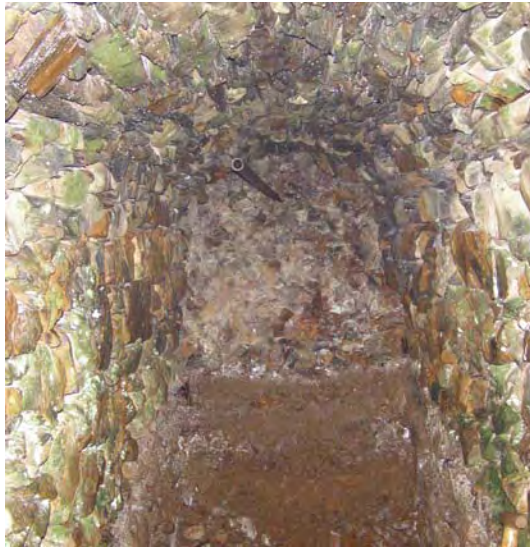
The scaffold pole can be seen protruding from the blockage.
