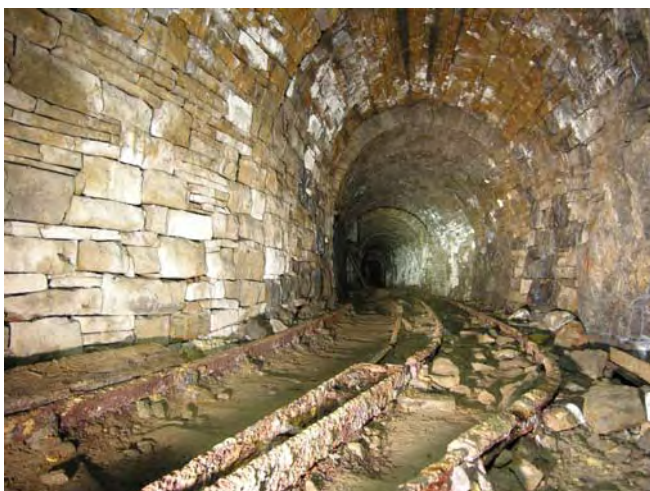
Twin railed service tunnel beneath the Brownley Hill Middle Vein stopes
