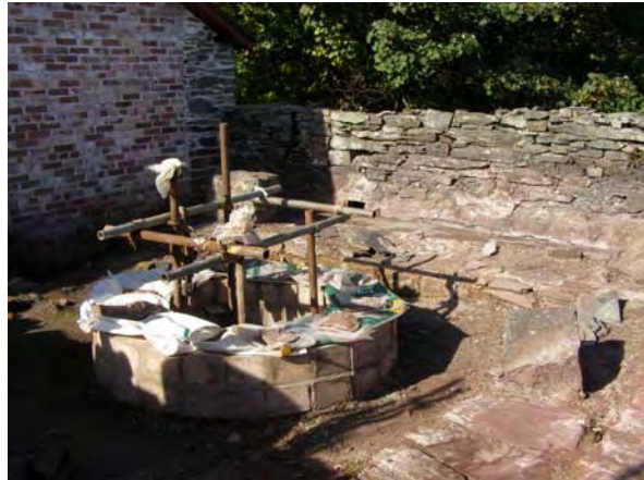
The top of the stack at Newland, showing the re-built furnace lining and revealing part of the base of the walls. One of the limestone blocks can be seen bottom right.
