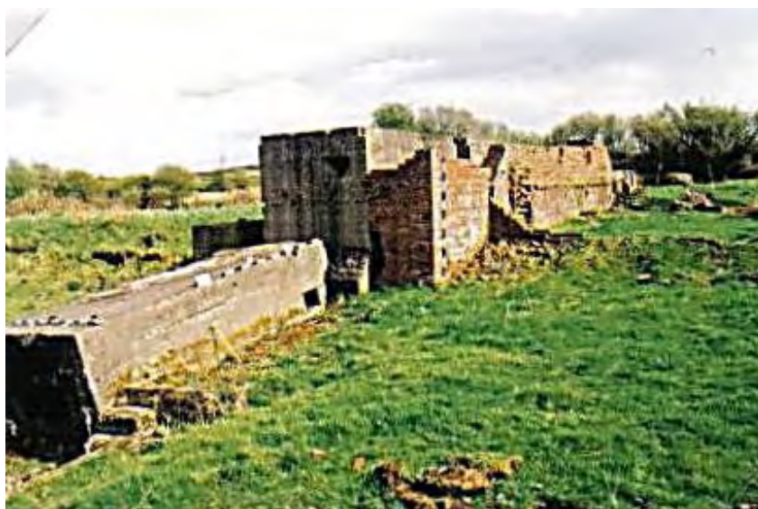
Base of Hathorn Davey engine at Violet Pit in 1996. Photo SCP Thomas
