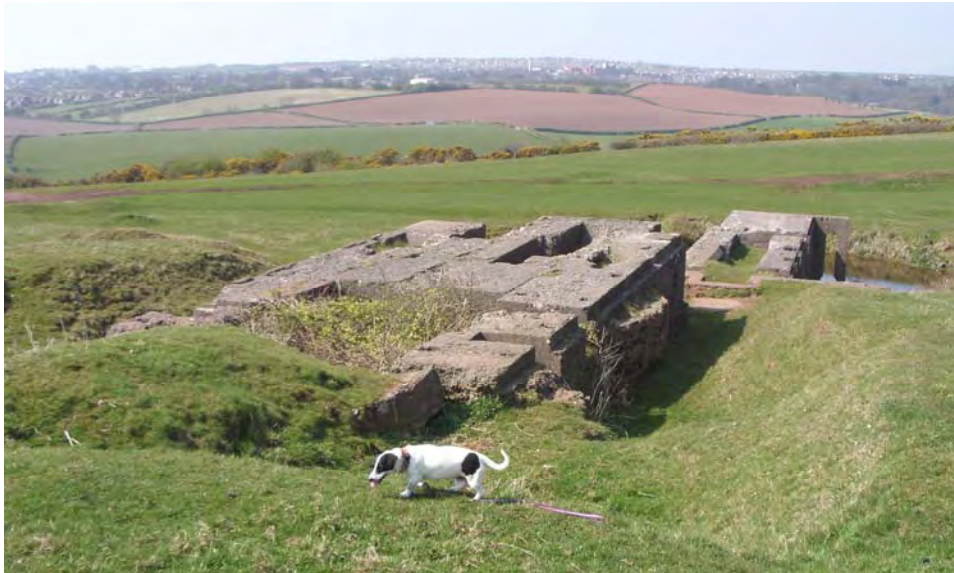
Base of Hathorn Davey engine at Yarlside No 11 pit. Photo P Sandbach
