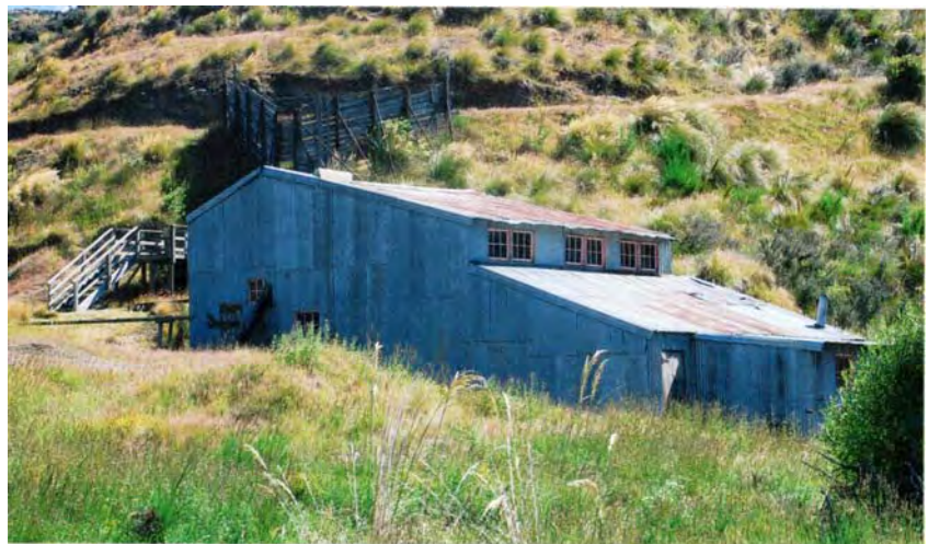
Gold Point Battery (Callery Battery). Deepdell Creek. Macraes. Battery treated gold and scheelite. Tramway and hopper can be seen to the rear.
