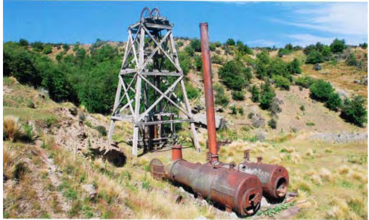
Golden Progress Mine. Original headgear from the 1930s. Australian timber. Two boilers still in situ. Shaft 200 feet deep.
