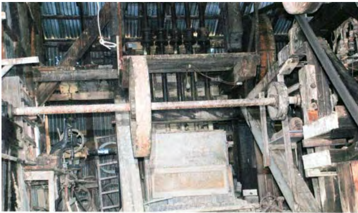
Five head stamps, powered by waterwheel, later by a 16hp Tangye Kerosene engine.
