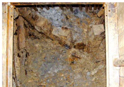
The work face, 17 th October 2010
