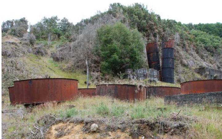
Snowy River Battery from the sands disposal area
