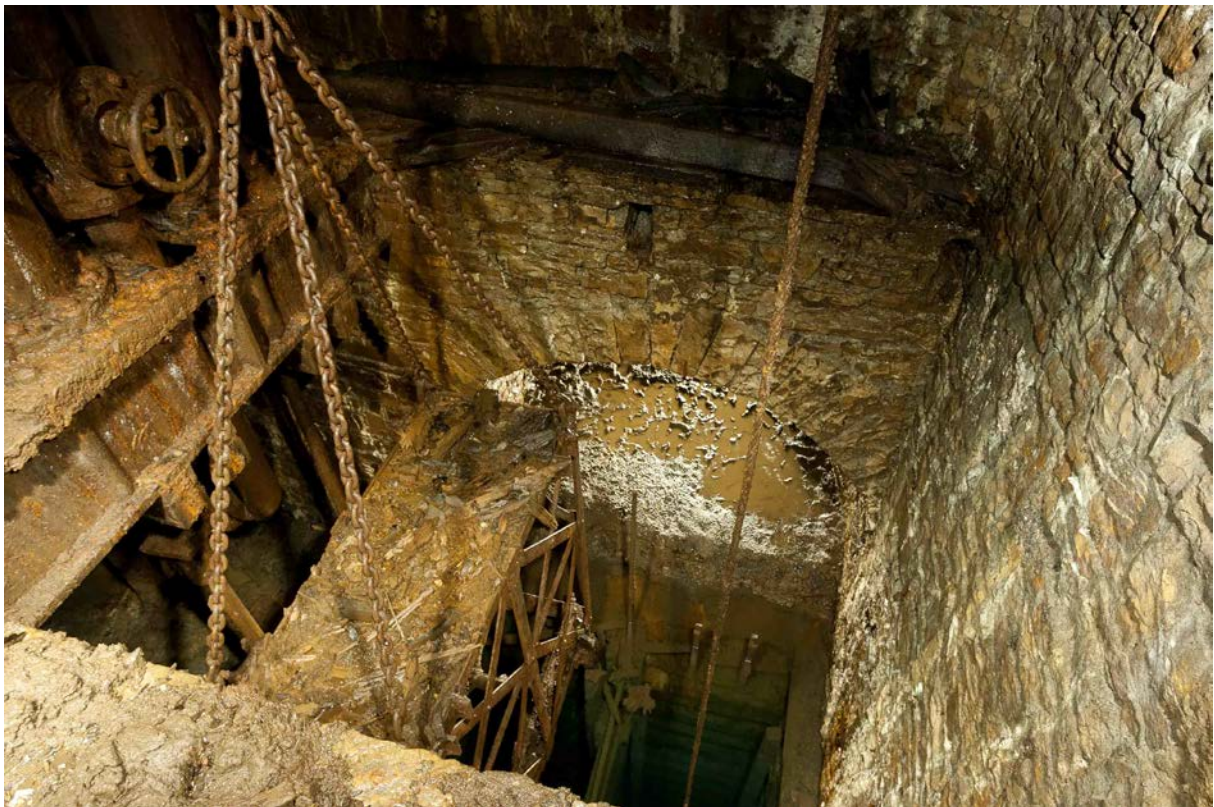
Shaft and cage in Sir Francis Level. Photo Chris Cowdery
