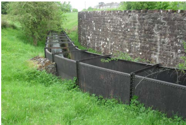
This iron trough was made to carry the beck over broken ground at High House mine in the 1880's.
