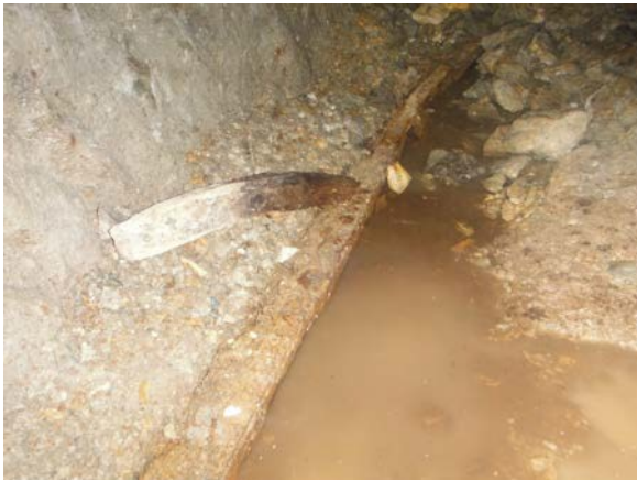
Wooden rails with iron capping
