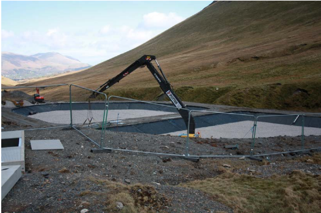
Looking over the top of the partially constructed ponds
