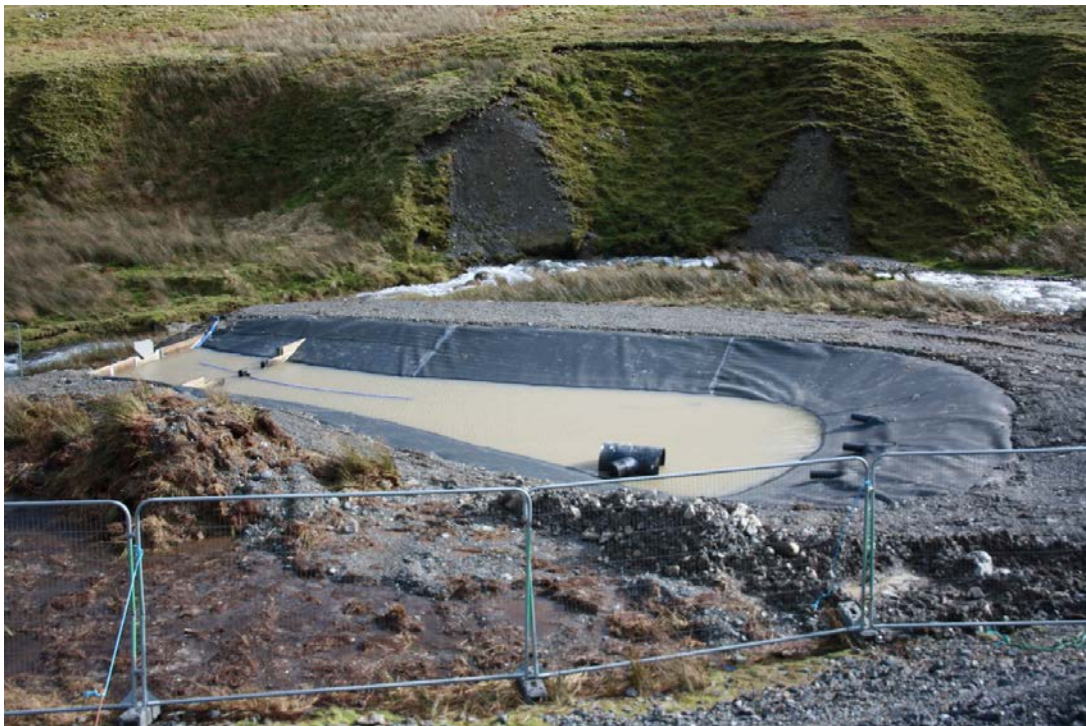
Constructing the finishing pond
