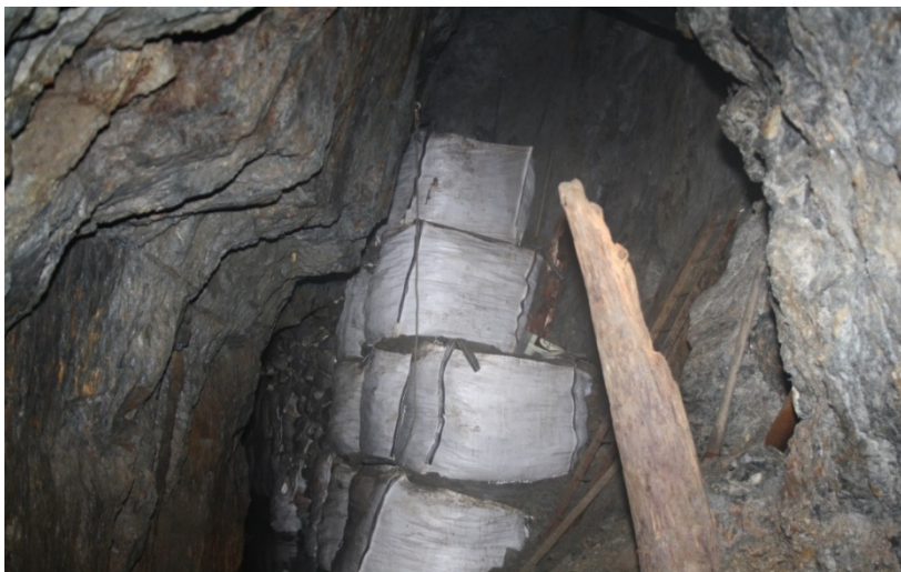
The pack wall is over 120 yards long and in places such as where we are now, nearly 20 feet high.
