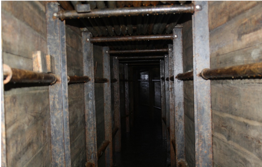
Looking back to the start of the second fall showing the kink in the steelwork. 19 sets have been installed
