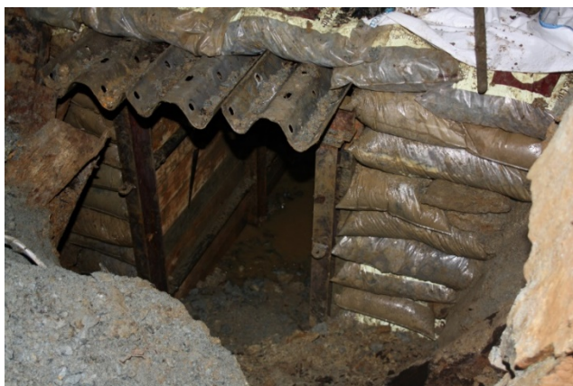
End of the third fall with the crash barriers installed.
