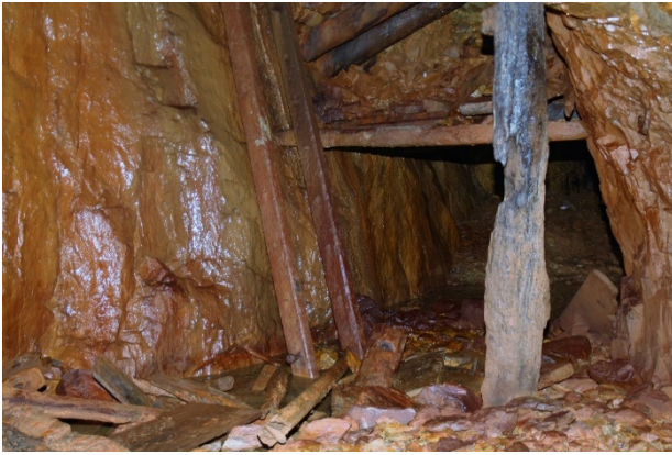
Bottom of the ladderway and ore pass
