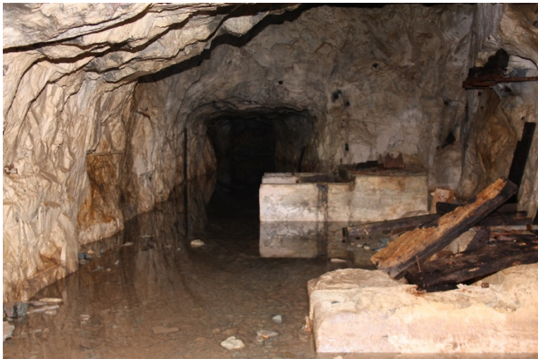
Two of the three concrete beds for the air compressors in Warsops Cross-cut where it enters the electrical switch room
