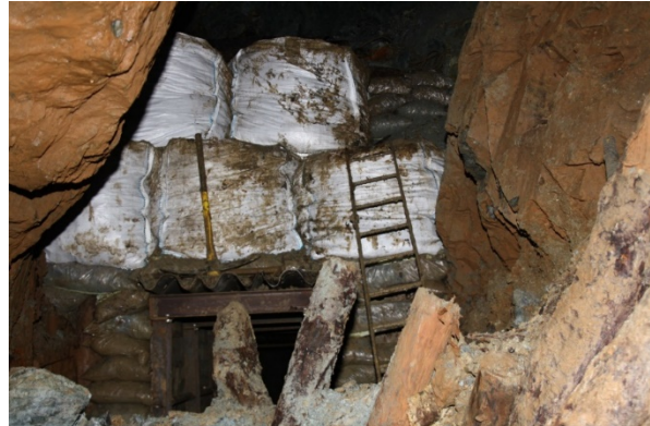
Building the pack wall above the end of the dig to stabilise the debris
