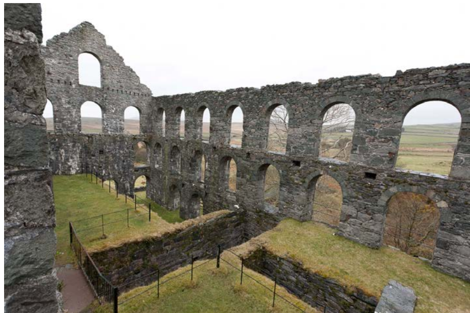
View inside the mill showing that the workings were on the three floors. The central pit was for a water wheel with the drive being in the culvert to the right with belts driving sawing and planning machines on the grassed area.
