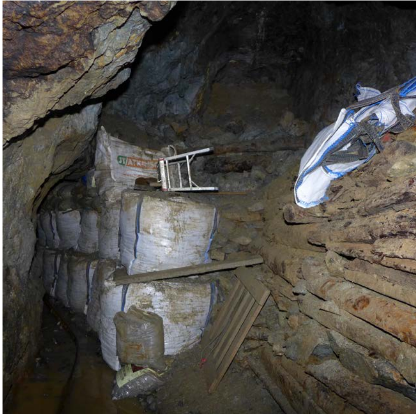
End of the bag wall looking out-bye, which is now 80 yards long and in places 15 feet high
