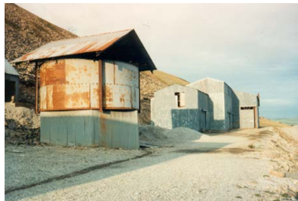
Primary crusher on the left, with the main processing plant behind
