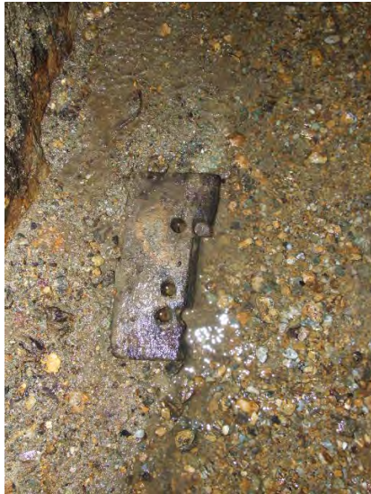
Sleeper in-situ- note the wooden peg
