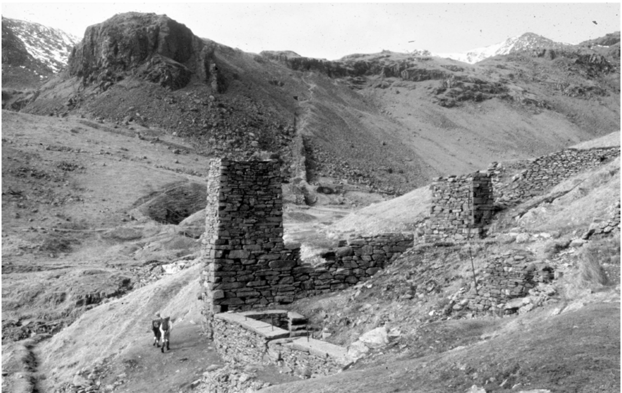
Old Engine Shaft wheelpit and Triddle incline, Coniston Coppermine
