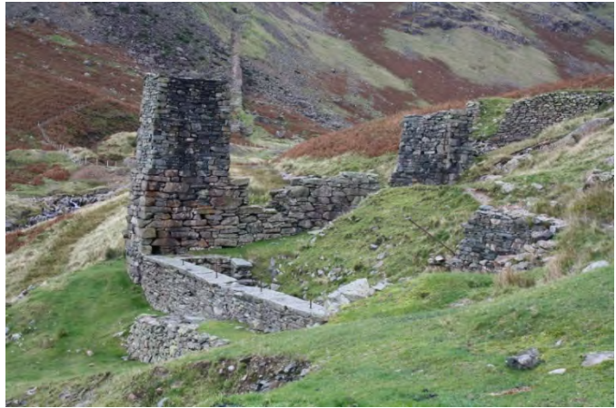
The Old Engine shaft wheel-pit & launder towers.
