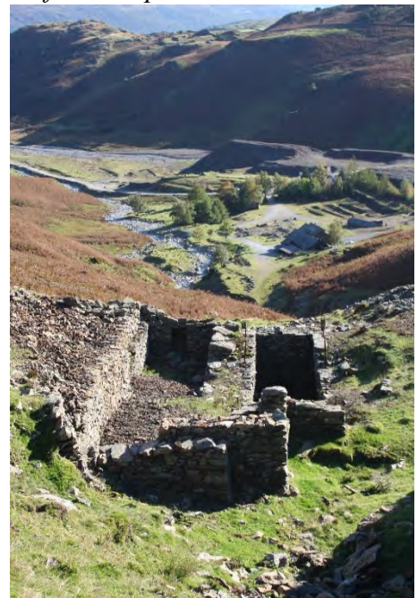
The Old Engine shaft wheel-pit & launder towers.
