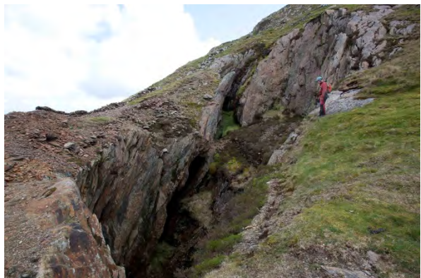
The stope where it has been worked through to surface
