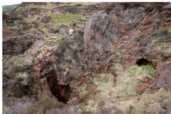
Shaft breaking surface in surface digging.
