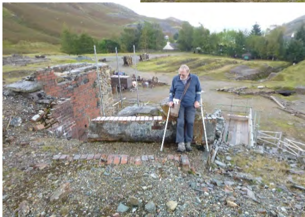
Ian Matheson, standing in the launder which carried the water from the upper waterwheel to the lower one next to the tower
