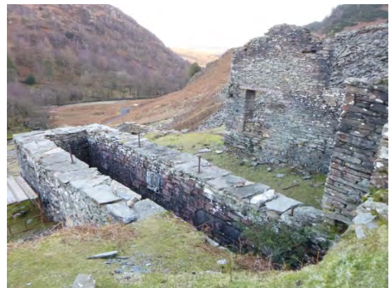
The capping stones on the top of the waterwheel pit have been replaced
