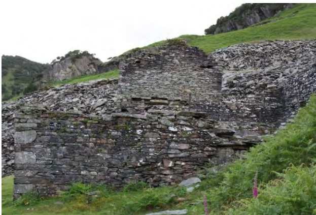
The collapse on the side of the waterwheel pit has been rebuilt
