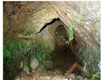
D (ii) - Inside Short Grain Low Level, a short collapse in unstable ground
