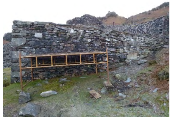
The collapse on the side of the waterwheel pit has been rebuilt
