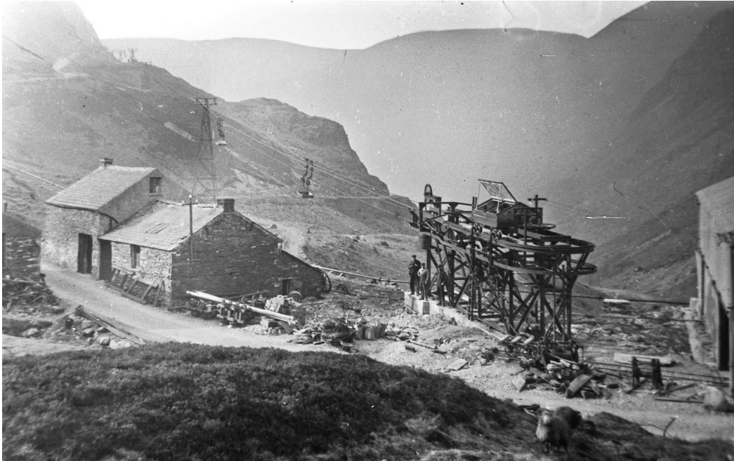
Aerial ropeways station at Honister House.
