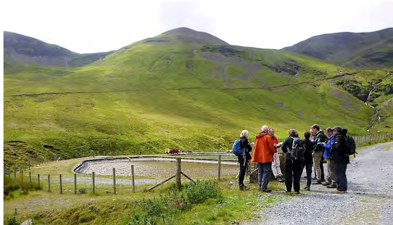
Down at the treatment plant
