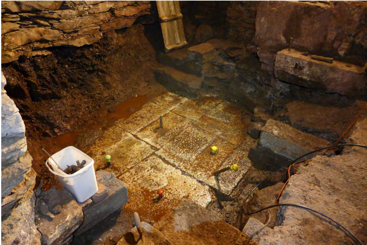
Blowing cylinder floor made of six dressed limestone blocks
