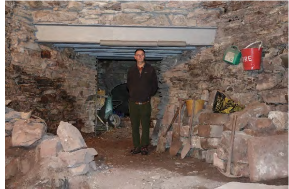
Current status of Blowing Chamber arch
