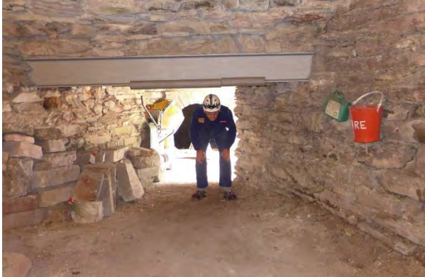
Blowing Chamber arch before work started
