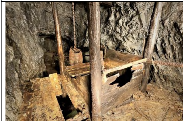
View showing how water was deflected into adit.
