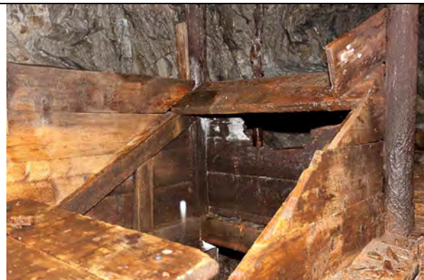
Frame and moveable trap door.
