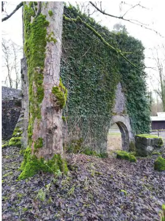
End wall of the incorporating mill
