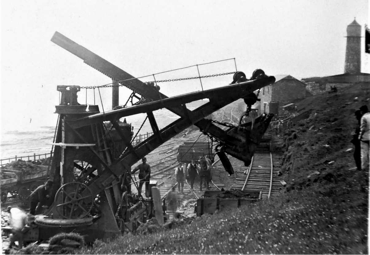
Steam Shovel working on Inner Barrier – SC
