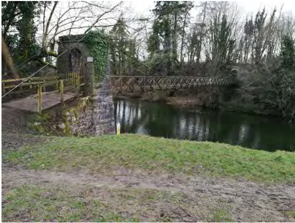
Footbridge looking from the east side of the river
