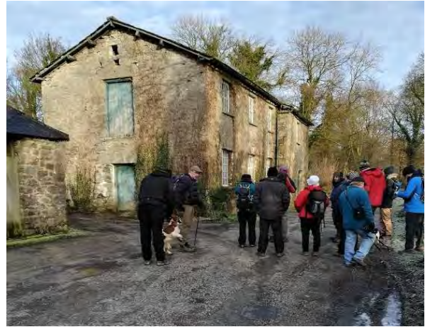
The turbine house
