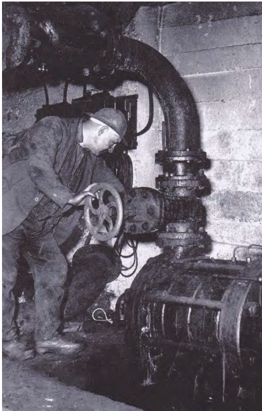
Underground at Moor Bank 1960 – Newspaper 1960s. The guy at the pump valve is sand filling a void
