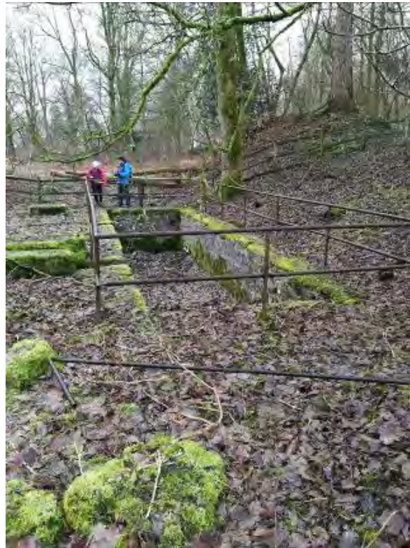
The turbine plant
