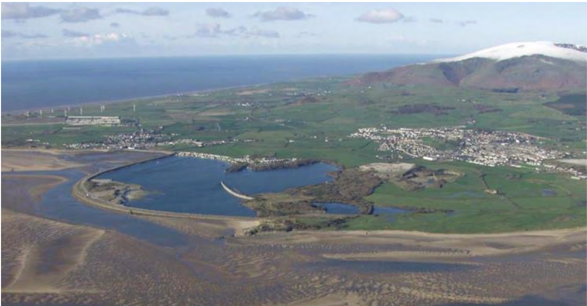
Hodbarrow Sea Walls from the air, 1990s – photo by Lawrence Hill
