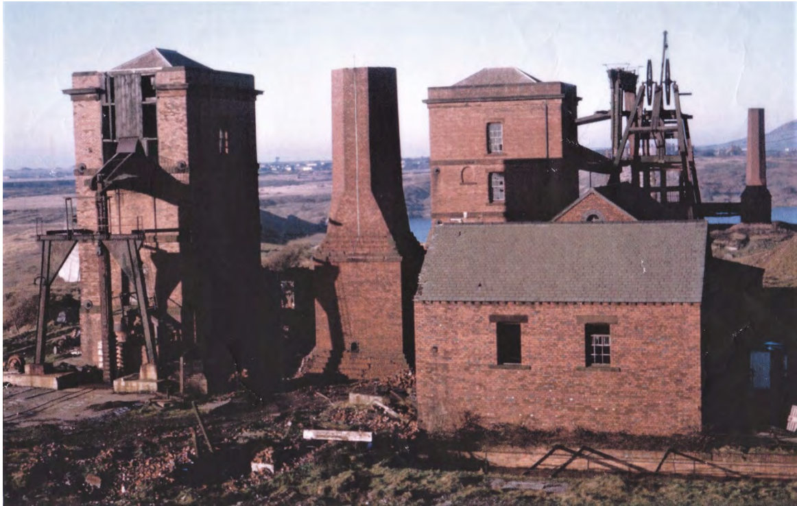
Remains of No 8 (Right) and No 10 (left) after closure – by Gilbert Scurrah
