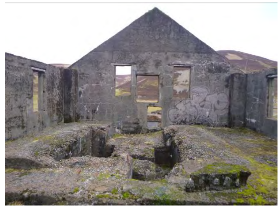
Winding engine house
