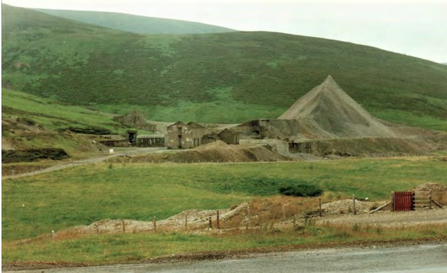
New Glencreif mine, where the buildings appear to be in better condition.
