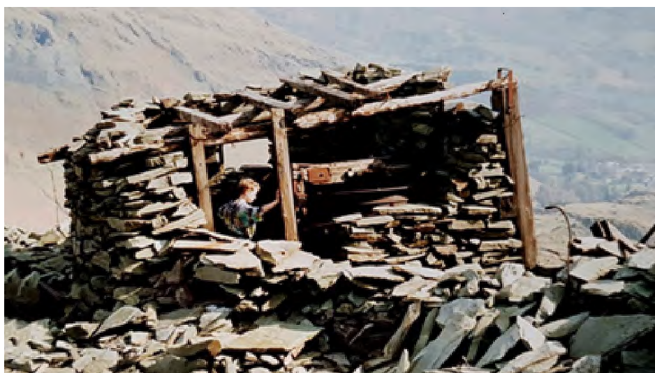
A photograph taken 20 years ago of the drum-house that controlled the inclined aerial flight that ran from the High Moss Head site down to the Saddlestone Bank. The incline carried slate ‘clogs’ (blocks) from which slates were manufactured in the riving sheds at Saddlestone.
