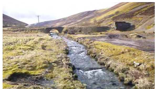
The remains of the smelter at Leadhills
