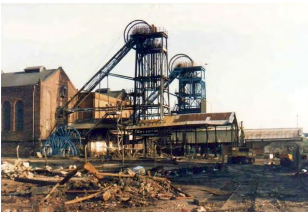
Photo showing demolition of Haig Colliery 1986/1987.
