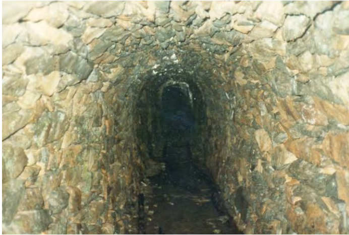
The stone arched level had wooden rail, of which there are remnants, and was driven in a straight drive.
