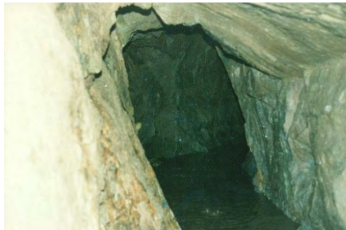
The stone arched level had wooden rail, of which there are remnants, and was driven in a straight drive.
