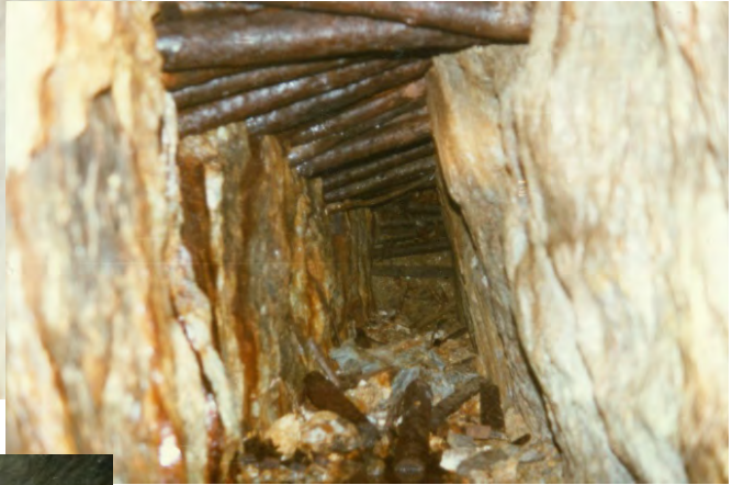
Timbering in the original level.
