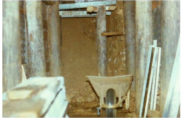
The front of the dig as we drove timber into the soft ground in front.
