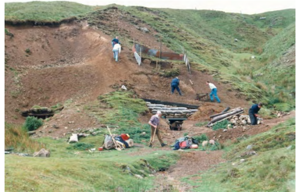
Material from the collapse was wheelbarrowed to back fill above the level.
