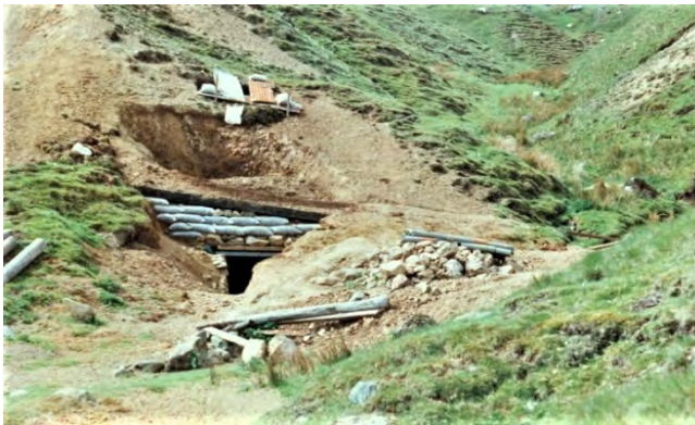
Restoring the entrance and note the hole above.
