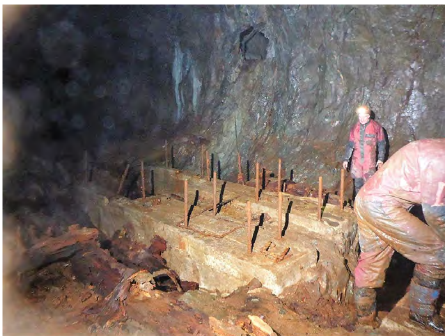
Engine beds, the access hole is visible upper centre of the picture.
