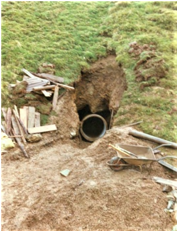
Pipe in position
