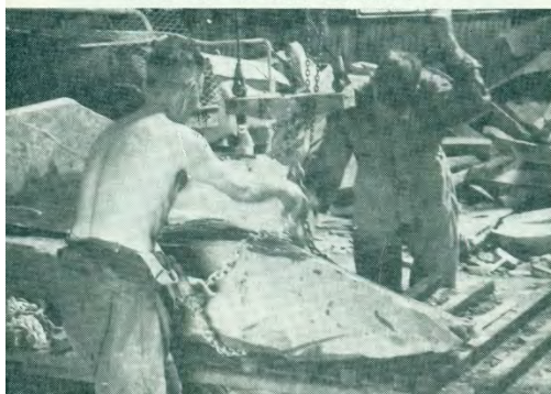
Honister green slate being prepared for the saw which cuts it into handy pieces.
