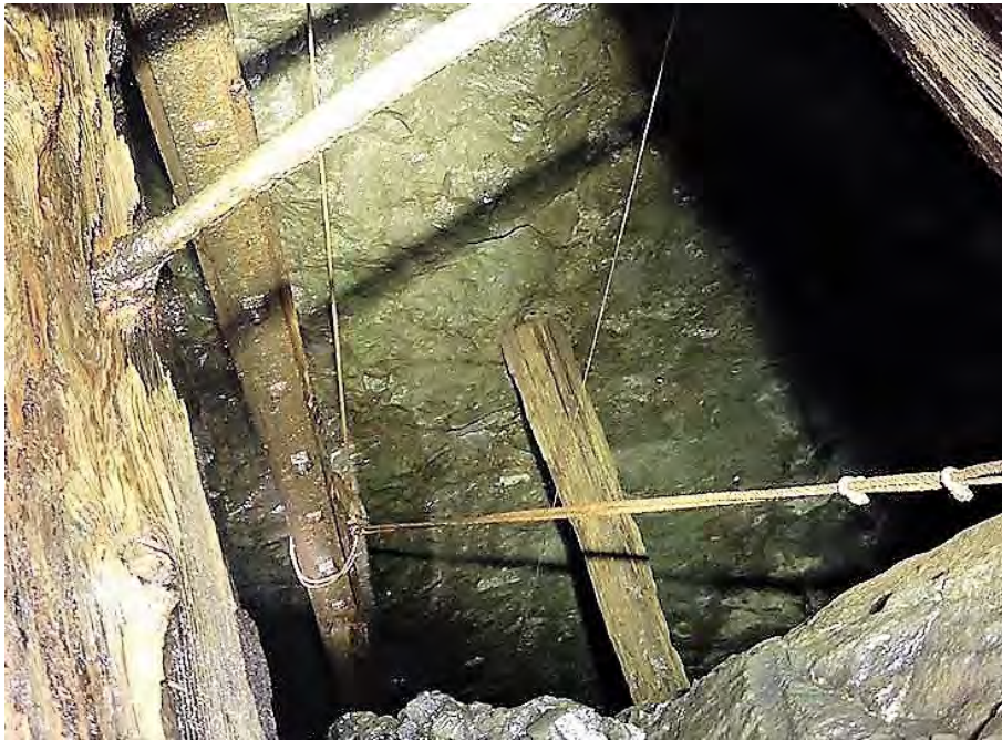
The supporting wires taking the strain. They were installed by CATMHS in 1991.
