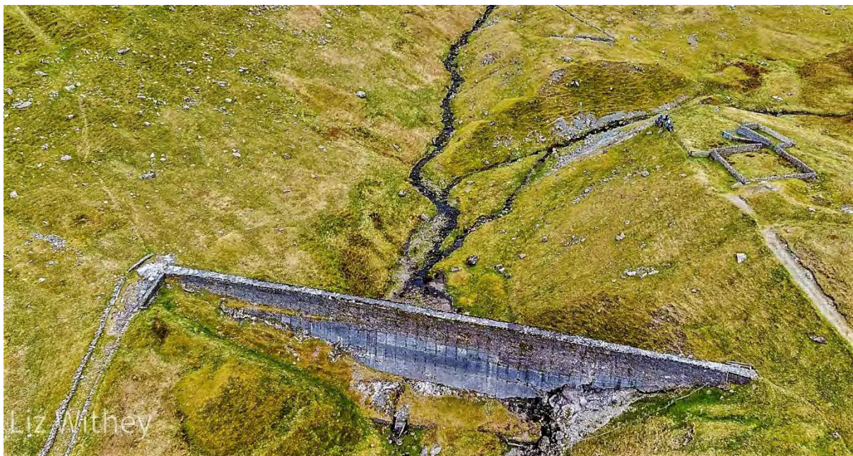
Drone image by Liz Withey showing the breach in the tarn above the sheepfold and the concrete dam with spillway to the left and the breach in the bottom right-hand corner.
