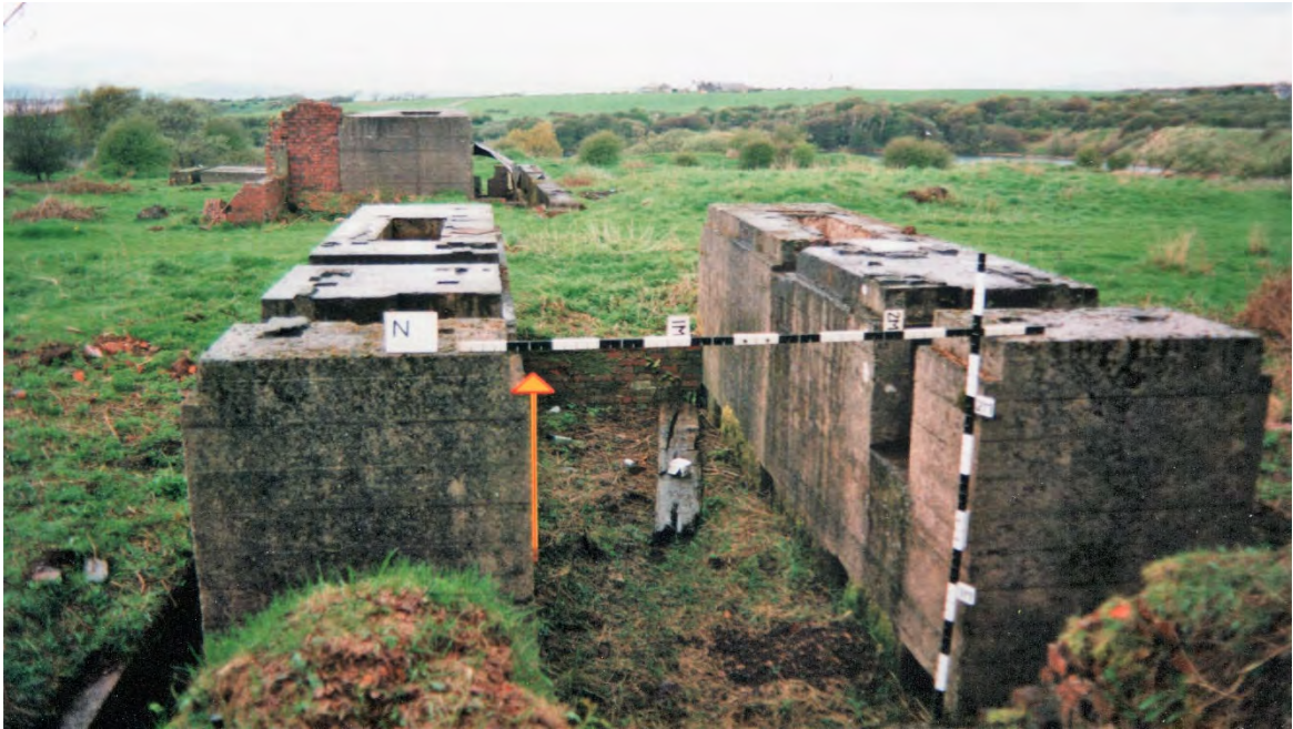
Base of Hathorn Davey engine at Violet pit.
