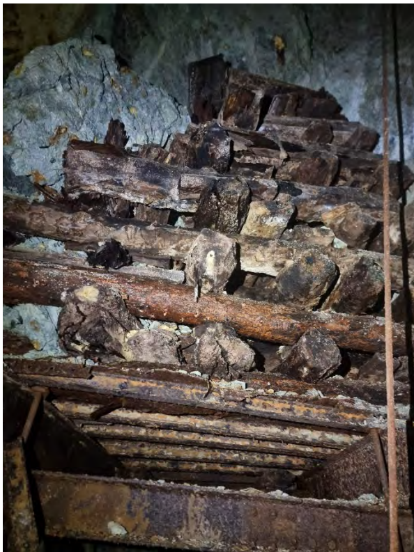
Figure 2: Crows nest 04/02/23 (left) and 18/02/23 – images from the same angle are not available, but the instability on 18/02/23 is apparent.
