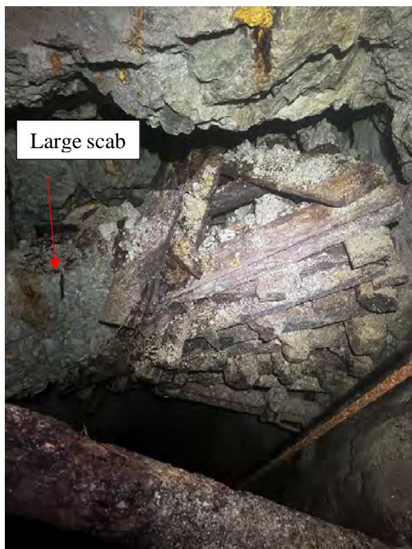
Figure 2: Crows nest 04/02/23 (left) and 18/02/23 – images from the same angle are not available, but the instability on 18/02/23 is apparent.
