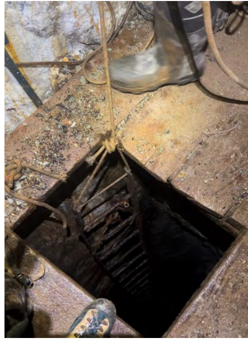
Figure 1: Removal of part of the buckled and distorted ladder close to the base of P8 (left) and lowering of damaged ladder from the boulder (right)
