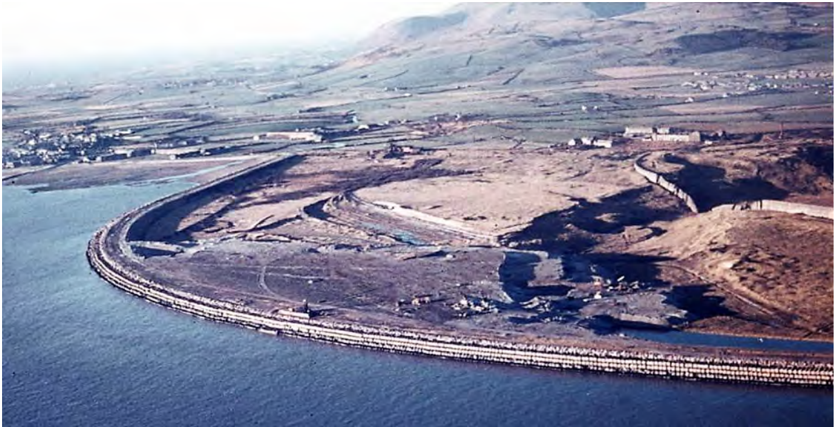
The Outer Barrier, the Broken Ground and the collapsed Inner Barrier.
